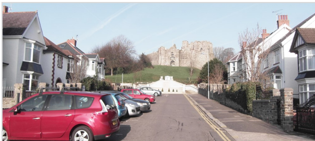
Views up Castle Avenue with stairs into castle grounds
