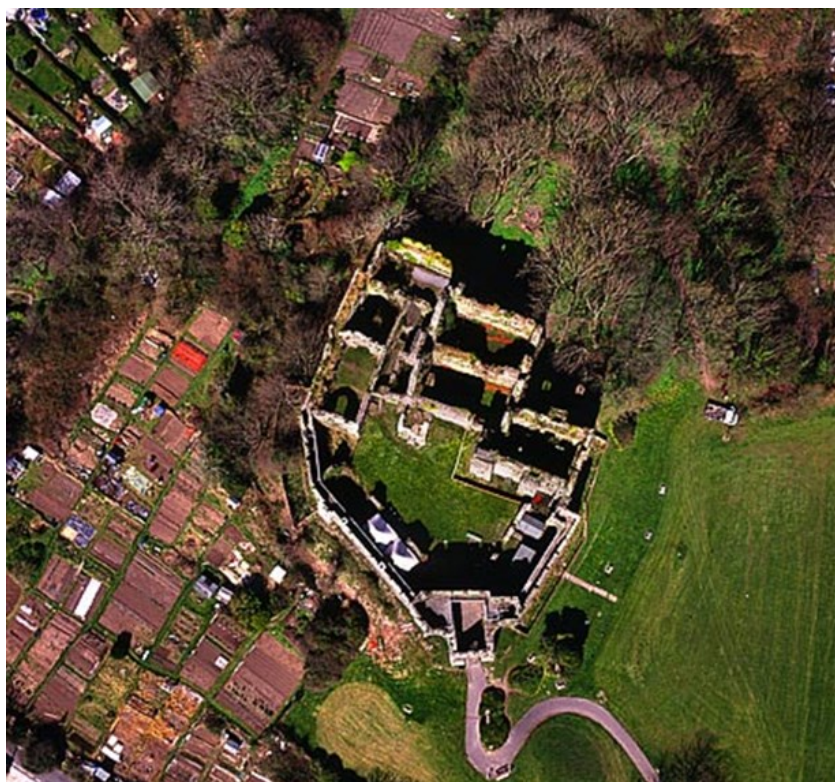
Aerial view of the castle showing its grassed hill setting, the screening belts of trees and the allotments site.
