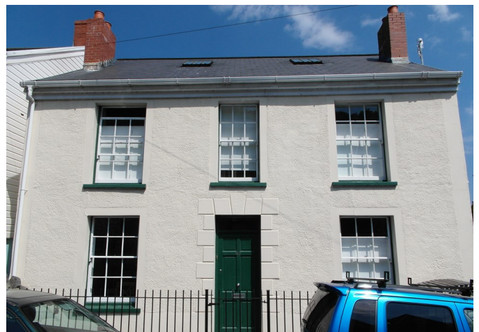
A good example of renovation of a residential dwelling on Overland Road.
