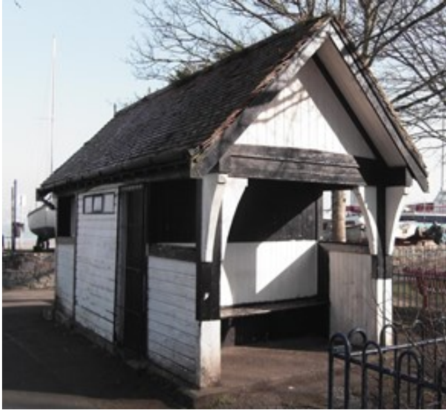
Shelter, Southend Gardens
