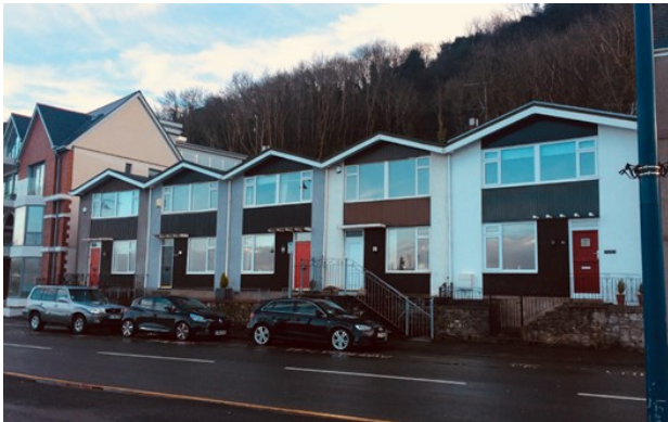
Inappropriately styled development that does not integrate with adjoining buildings can negatively impact upon the heritage townscape
