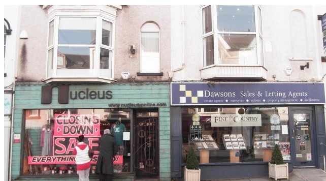
Inappropriate shopfront design and materials detracts from the visual qualities of the Conservation Area
